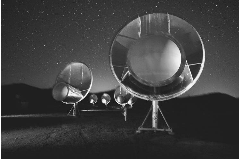
Figure 12.7. The Allen Telescope Array in northern California is the most sophisticated SETI project ever. It will deploy 350 radio dishes working together with a wide field of view to examine sunlike stars for artificially produced signals that would reveal the presence of extraterrestrial intelligence.
